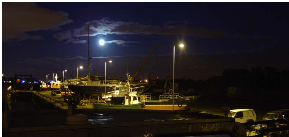
Figure 2: Purpose built boat yard with hoisting facilities.
